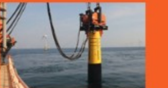
FREE HANGING INSTALLATION WITH VESSEL ON DP
